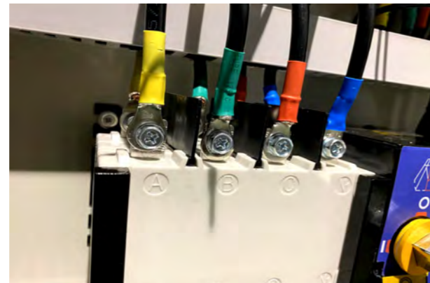
Dual Power Supply Wiring
